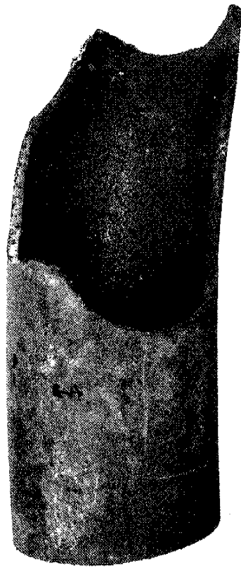
Figure 28. Rupture, blistering, and hydrogen embrittlement in 8-in. Schedule 80 carbon steel pipe.
